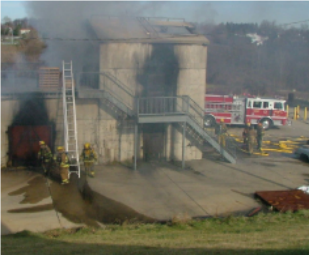
A structural firefighting building in use during a training evolution
